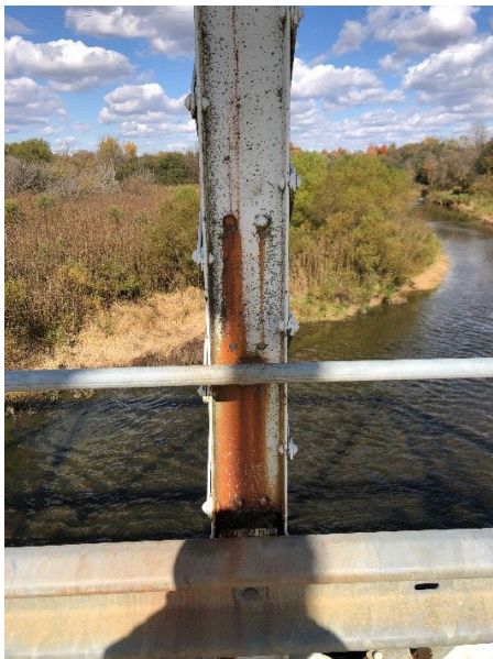
Figure 4: Photo of Corroded Beam on Blacks Bridge
