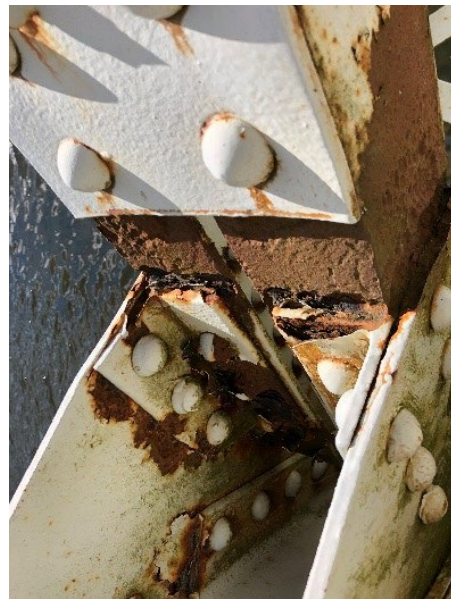
Figure 5: Photo of Corroded Joint on Blacks Bridge
