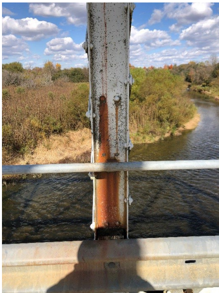
Figure 4: Photo of Corroded Beam on Blacks Bridge
