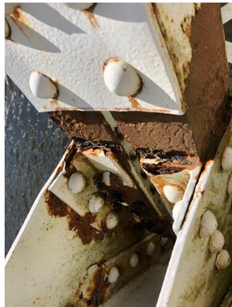
Figure 5: Photo of Corroded Joint on Blacks Bridge
