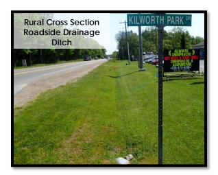
Rural cross sections typically consist of gravel or paved shoulders, and roadside ditches for stormwater management, and are typically used on higher speed roadways. While rural cross sections do not preclude the addition of sidewalks or streetscape elements, they are typically constrained by existing right of way limits.
