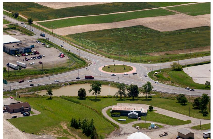
Traffic circulates counter-clockwise around the central island. Entering vehicles must yield to all traffic already in the roundabout
